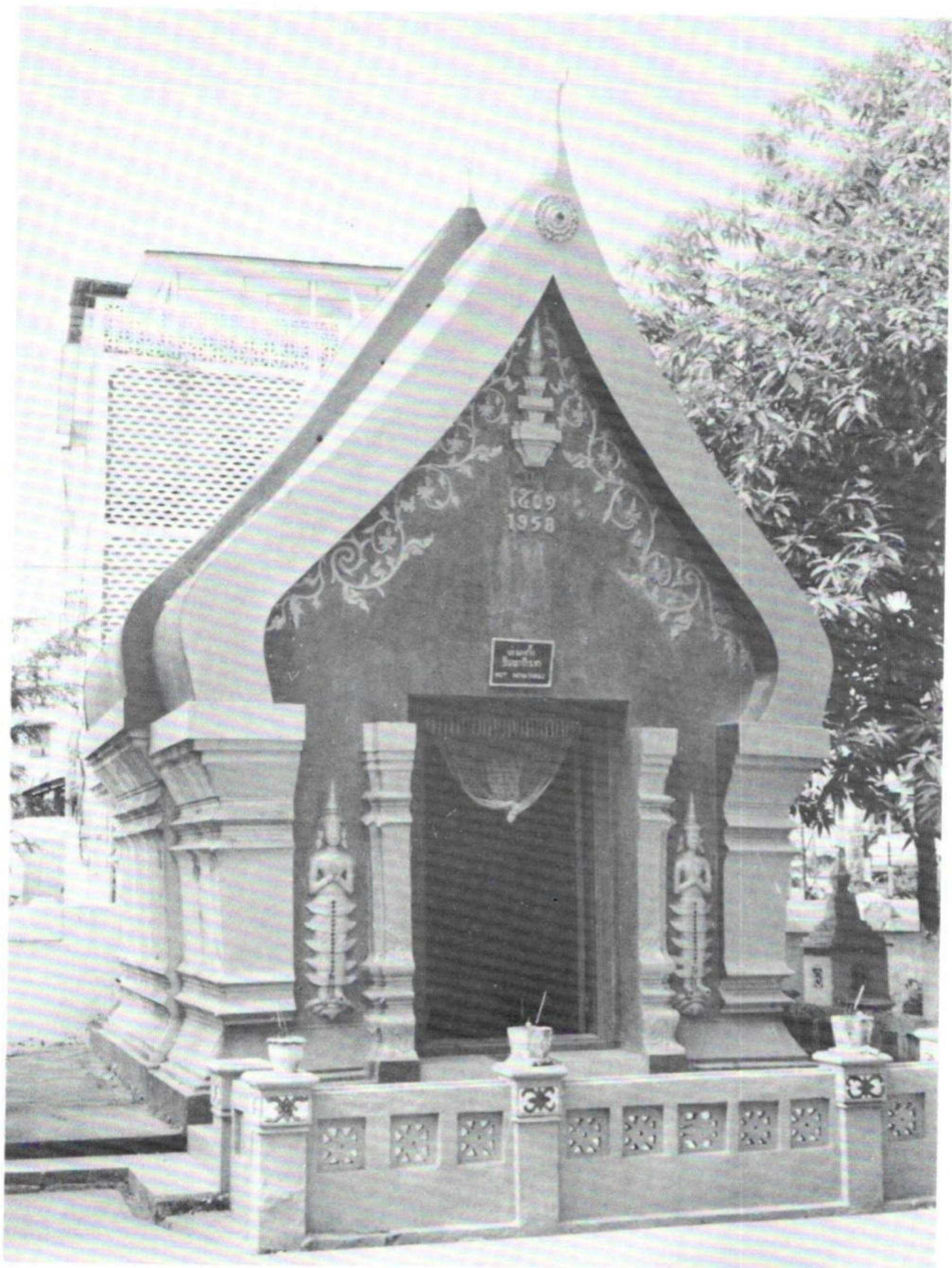
- ອຸບມຸງ ບ່ອນສະກິດພະເຈົ້າອິນທາທິຣາຊ THE NICHE BUILDING FOR THE INTHATHIRAJ Buddha Statue
